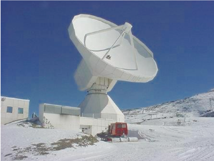
Fig. 1.22. The 30-m telescope on Pico Veleta was designed for observations in the millimeter range of the spectrum. This telescope, like all millimeter telescopes, is located on a mountain to minimize the column density of water in the atmosphere
